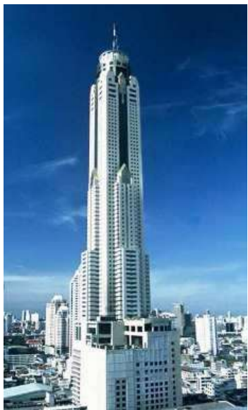
BAIYOKE SKY HOTEL Currently the tallest building in Thailand - M.E.P. -
