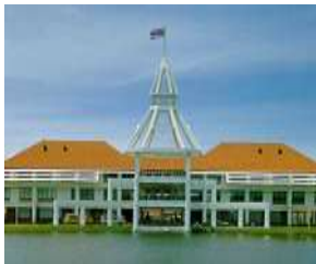
THAMMASAT UNIVERSITY (Rangsit Campus) - Main Admission Office Building - Lecture Building I - Lecture Building III - Lecture Building IV - Faculty of Engineering Building (Int.) - Library Building (Bangkok campus) - Laboratories - Multi-Purpose Building (Bangkok campus)
