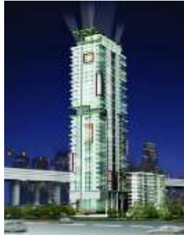
INTRO BY RASA Condominium - M.E.P -
